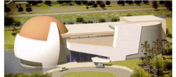
Entrance to Dekelbom Science Center
